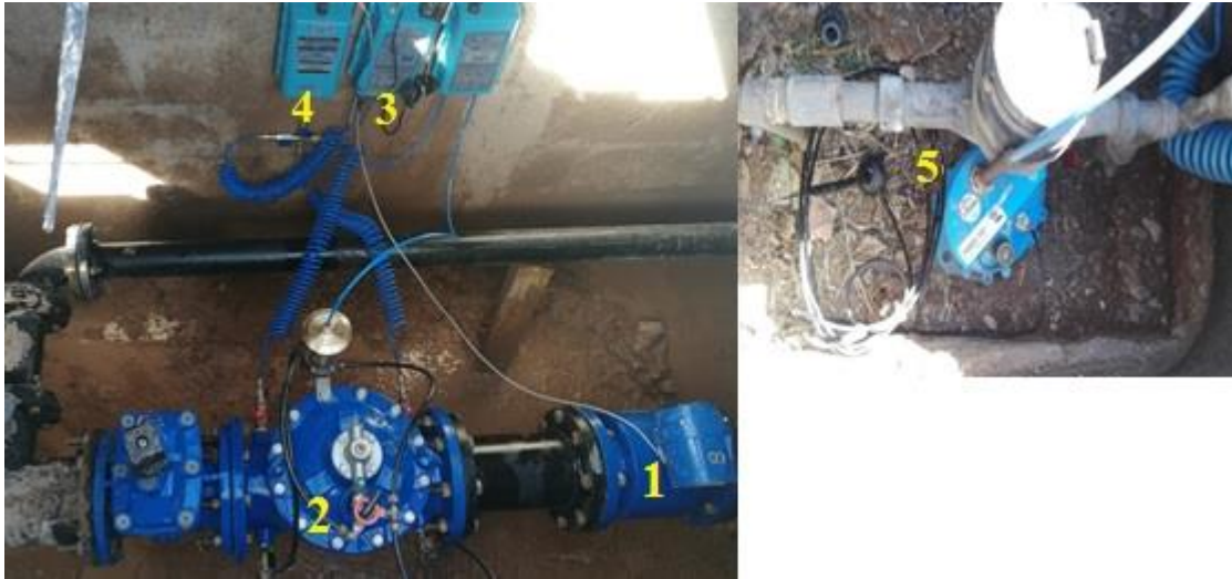
Fig. 2 Real-time instrumentation for pressure management in the city of Chihuahua, México. 1. Electromagnetic flowmeter. 2. Pressure regulating valve (PRV). 3. PRV controller with GPRS communication. 4. Multilog, advanced data logger with integral GPRS telemetry. 5. Multilog, advanced data logger with integral GPRS telemetry at a critical point.
